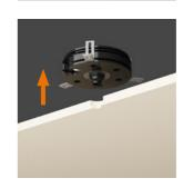
MAINTENANCE Cut the plaster and remove the luminaire by unscrew the screws
